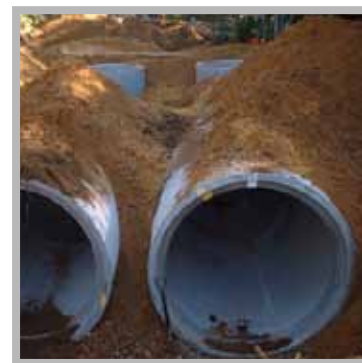
End entry manholes
