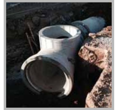
1200mm side entry run being installed
