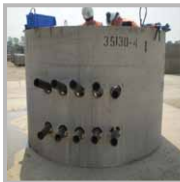
2100mm chamber with pipework cut out in chamber wall
