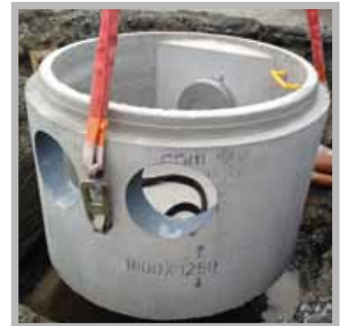
1800mm sealed chamber complete with Optimum Hydro-Brake®
