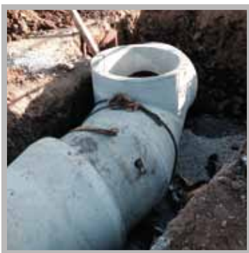
900mm off 900mm mid entry manhole
