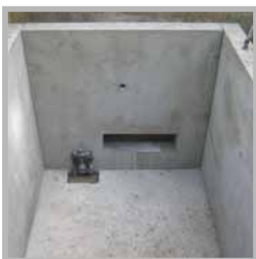
Once-piece chamber with inlet and outlet holes
