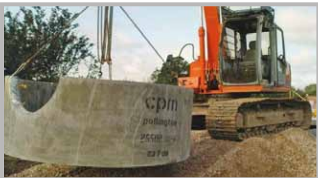
2550mm sectional installation, base chamber complete with half formed hole for 750mm pipe
