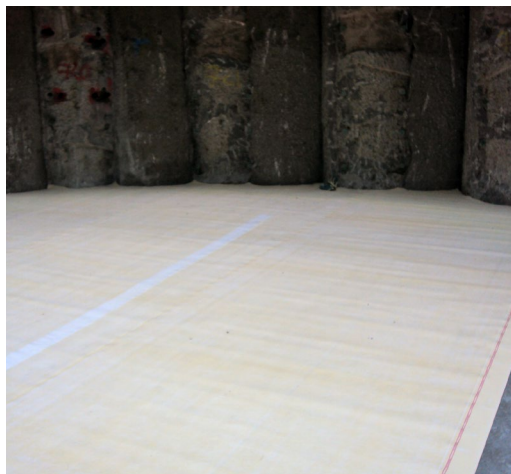
Fully bonded SikaProof®A-12 waterproof membrane system
