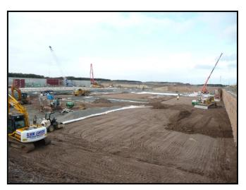
TerraConsult was employed by Birse, the Principal Contractor for the construction of Vault 9, to provide advice on the construction of the engineered containment lining systems and drainage. TerraConsult are one of the UK's leading experts in the use and practical application of Bentonite Enhanced Soil Lining materials and geomembranes for containment engineering.
