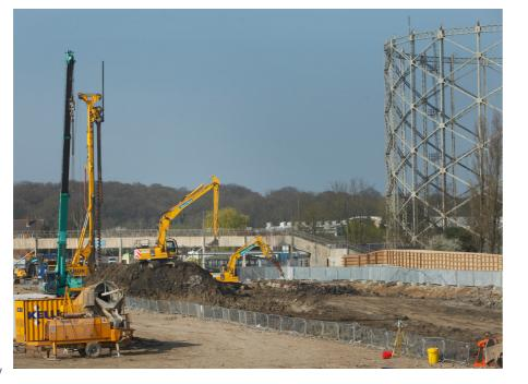
deep basements. 61,000m<sup>3</sup> of the overall excavation volume was determined to be potentially contaminated and was subject to selective excavation, sorting and classification in accordance with the remedial strategy. Approx. 24,500m<sup>3</sup> of this material subsequently underwent treatment utilising bioremediation and soil stabilisation / solidification techniques. All the treated soils were retained on site and re-engineered in accordance with the agreed Earthworks Strategy.
