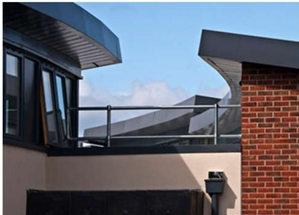
Eaton Valley Primary School, West Bromwich Structural and Civil design for a new Primary School. General ground improvement techniques were utilised for the foundations with a number of environmental initiatives.
