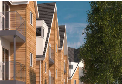
Sidcup, London Care Village. Structural engineering for the sub and super-structure designs, incorporating a complex roof structure of this 50 unit scheme.
