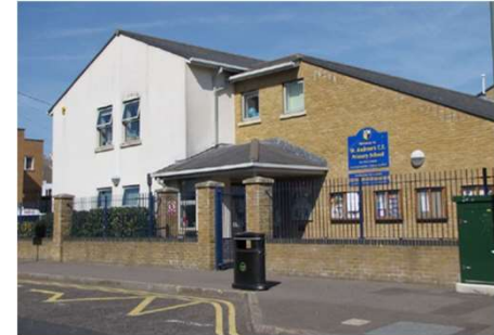
St Andrews School, Hove Structural and Civil design for a new build primary school. project consisted of a loadbearing masonry structure over 2 storeys.
