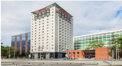
IBIS Wembley, Refurbishment Pinnacle instructed to carry out the detailed design of new front of house modifications to the multi storey building. Majority of the works involved new customer vertical circulation routes around the reception area and to the breakfast rooms on the first floor.
