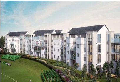
Canterbury, Kent Development of 60 Ortus flats with improvements to the cricket ground including landscaping, re-organisation of the supermarket and formation of a new vehicular access.
