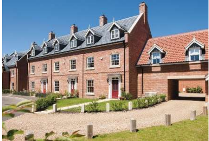
Soham, Cambridgeshire 96 plot residential development, statutory approvals and Anglian Water SuDS adoption.
