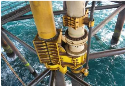
Structural Visual Inspections
