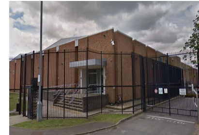
IRM Slough London Structural and civil engineers for a US client entering the UK market and supporting them on their first acquisition. Scheme involves the fit out of 3 new halls, plant support gantries over existing roofs, and new office block extension.
