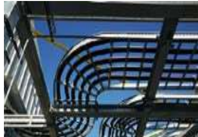
US / EMEA Concept Design Developing EMEA concept design model for large US client rollout. Scheme design has been in Level 2 BIM with full coordination with the MEP and Architectural teams.
