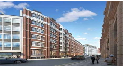
55 Newman Street, London Pinnacle carried out an extensive feasibility assessment of the current 6 storey office building to convert to a new boutique hotel for an overseas client. This included major structural works such as retention of the facades to allow the internal frame to be demolished, a new double basement dig and a new structural frame installed, including adding two additional storeys to the building.
