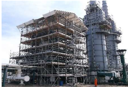
Gas Terminal Inspections
