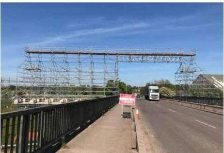
Lyndon SGB provided a large overhead line protection scaffold for main contractor Babcock International on behalf of the client National Grid on the Hams Hall ZF/ZFA Route – part of the exciting "once in a lifetime" HS2 rail infrastructure project. The purpose of the scaffold was to allow for the safe diversion of the existing overhead lines and installation of new lines – which will provide clear access for HS2.
