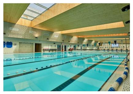
Seven of the rooflights, were positioned over the 50 metre swimming pool, adding an abundance of natural light, with special sun protective glazing to eliminate overheating. A special coating was applied to the aluminium profiles to protect them from corrosion within the chlorine environment. The rooflight, an 18m x 6m trapeze shape, illuminates the atrium at the flagship of the school's sports masterplan.
